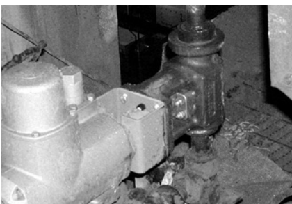
This ASME 4500 Class IRSVP convection vent valve was designed to handle extremely high pressure and elevated temperatures coming from the boiler.
