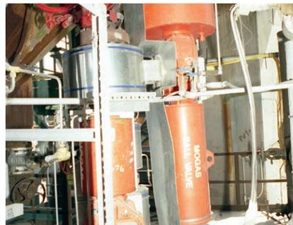
*These FCCU regeneration dump valves are still leak-tight after 60 months in 1400° F (760° C) service. Prior to the MOGAS metal-seated ball valves, the previous record was 3 months before lock-up or leakage occurred.*
