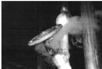
*Continual stem leaks from globe valves allows plant efficiency to decrease and maintenance costs to rise.*
