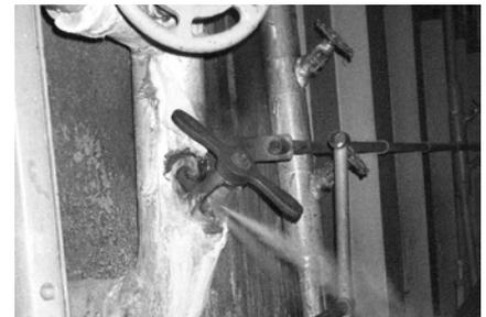
*The hazardous effects of high pressure wiredraw and the breakdown of torque seated sealing can create safety concerns and jeopardize the effectiveness of power generation.*
