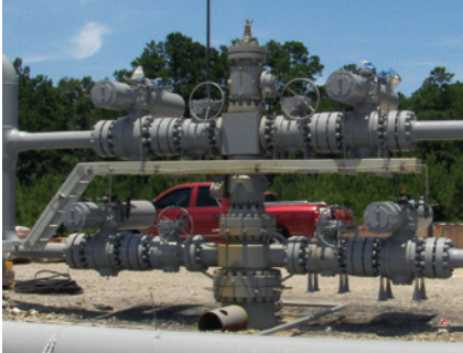
These FlexStream-designed valves are installed in a gas storage (salt cavern) facility. The valves have the unique capability to control pressure letdown in both the Cavern Fill and Cavern Withdrawal modes.
