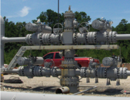
These FlexStream valves are installed in a gas storage (salt cavern) facility. The valves have the unique capability to control pressure letdown in both the Cavern Fill and Cavern Withdrawal modes.
